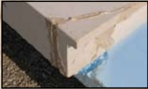
3 Reattaching stone with Extreme™ epoxy
