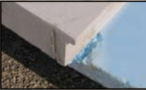
4 After grinding off excess surface epoxy
