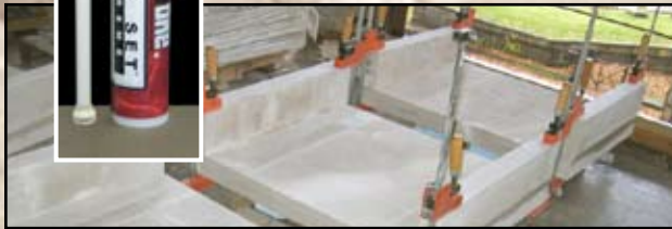
Anchoring and bonding large limestone assemblies using the EXTREME™ Epoxy
