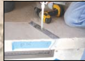
Crack injection gel system
