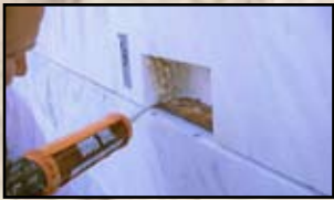
1 Applying Extreme™ epoxy
