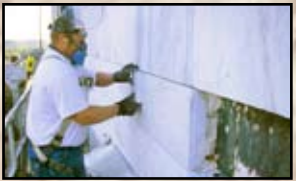
2 Positioning marble epoxy
