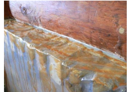
C. Work on project – paint or stain
