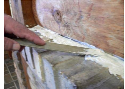
A. Apply Rubber Mask to substrate
