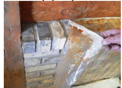
D. Remove Rubber Mask and plastic from substrate - no mess on adjacent surfaces
